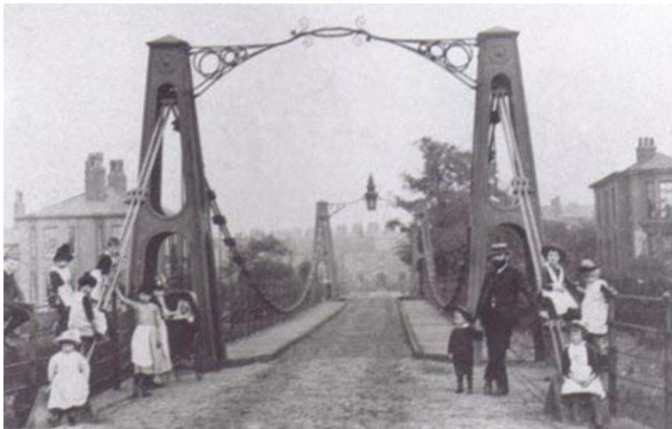
The Rebuilt Broughton Suspension bridge in 1883 (Photo credit: Richerman / Salford Local History library / Wikipedia)
